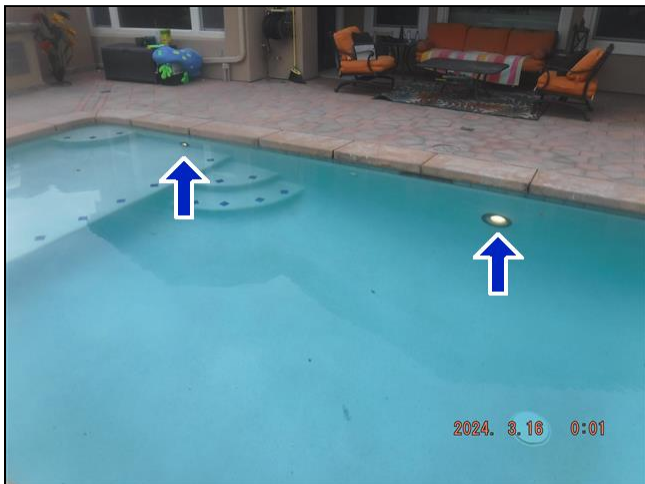
11.11 Item 1(Picture) Pool lights
