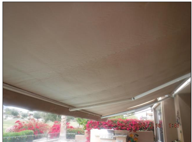
10.5 Item 2(Picture) Awning
