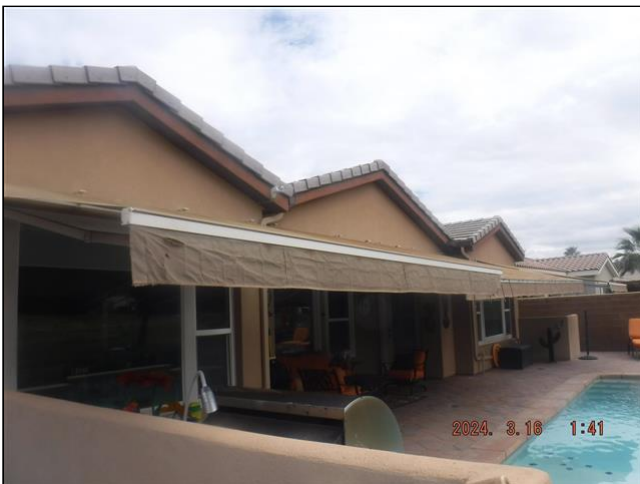
10.5 Item 1(Picture) Awning
