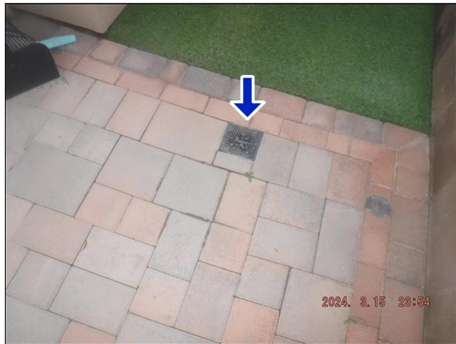
3.11 Item 2(Picture) Exterior plumbing drain
