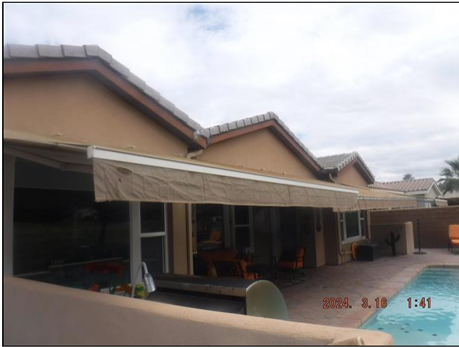
10.5 Item 1(Picture) Awning
