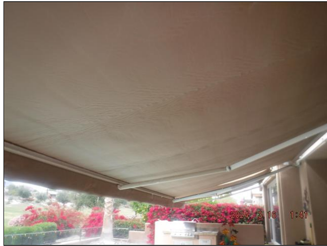
10.5 Item 2(Picture) Awning
