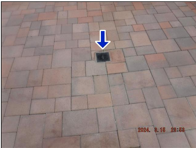
3.11 Item 1(Picture) Exterior plumbing drain
