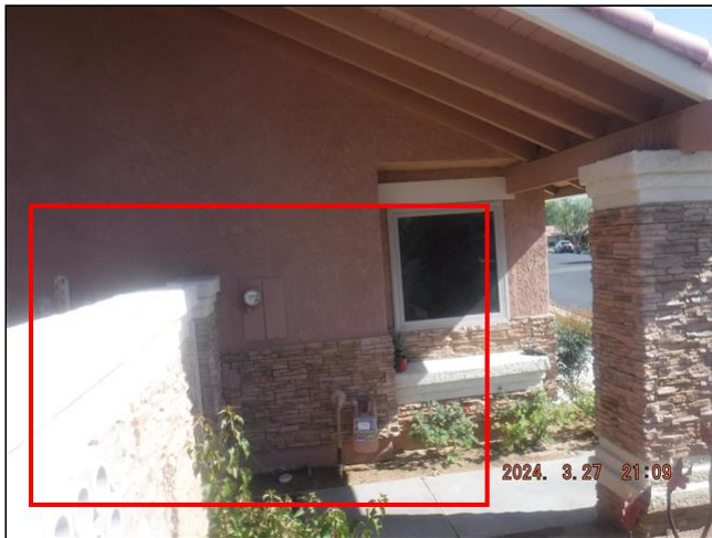
3.8 Item 2(Picture) Location of gas odor detected
