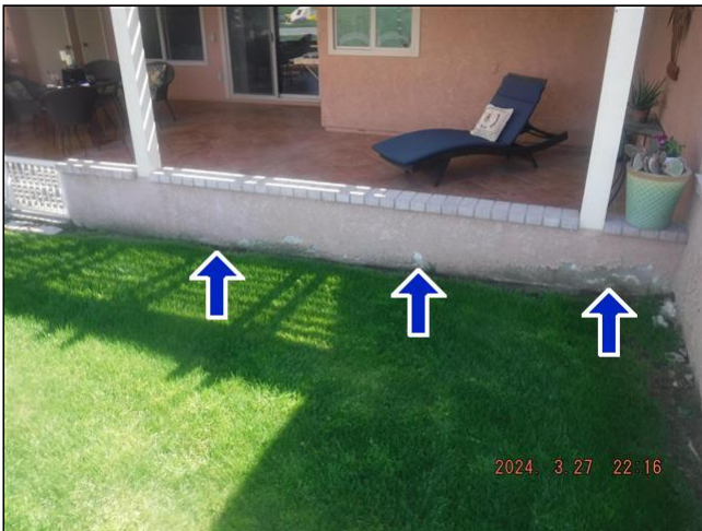
1.4 Item 1(Picture) Patio block wall
