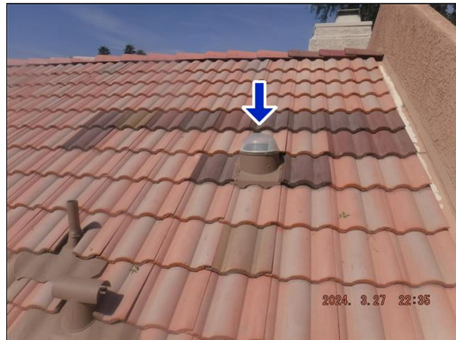
10.3 Item 2(Picture) Skylight
