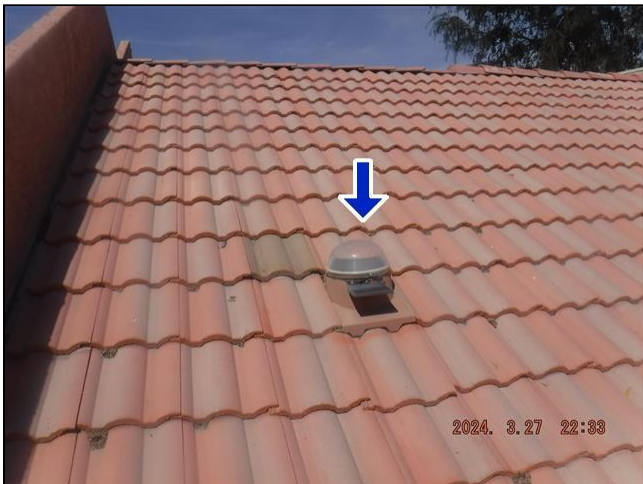
10.3 Item 1(Picture) Skylight
