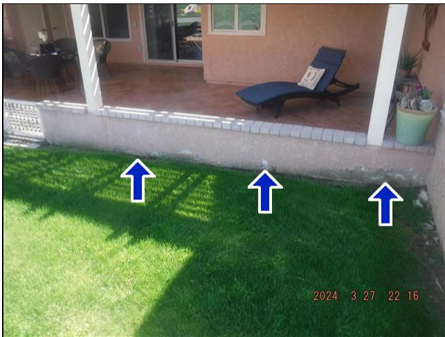
1.4 Item 1(Picture) Patio block wall
