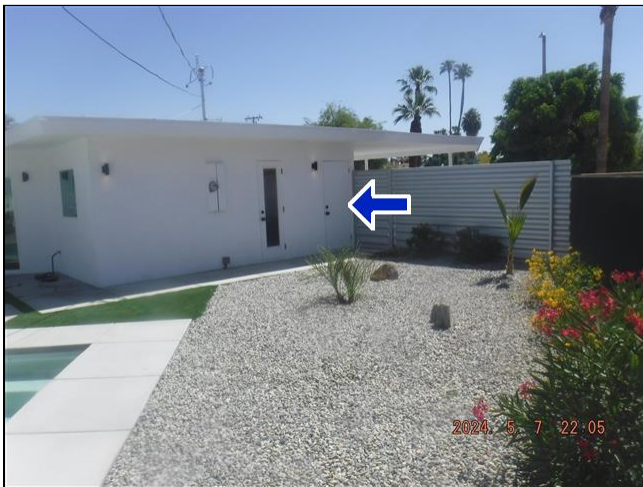
1.1 Item 3(Picture) Location of lock door
