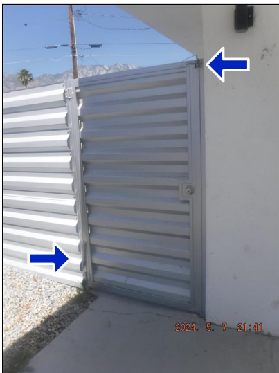
10.19 Item 1(Picture) Gate door
