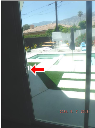
5.4 Item 3(Picture) Living room sliding door
