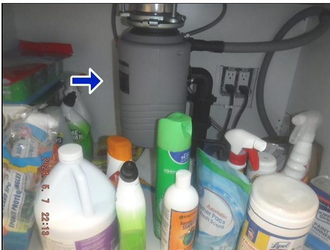
3.10 Item 1(Picture) Sink water valves location
