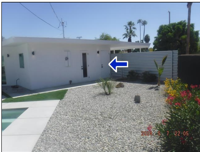
1.1 Item 3(Picture) Location of lock door
