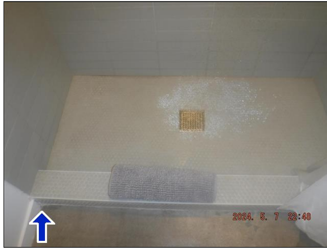
5.1 Item 2(Picture) Signs of water damage on wall
