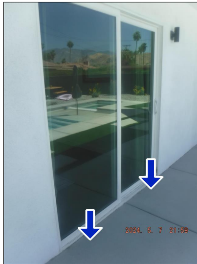
1.4 Item 2(Picture) Walkway height, or near to door threshold
