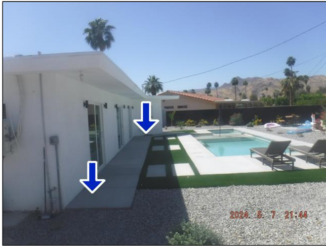
1.4 Item 1(Picture) Walkway slab slope back of home
