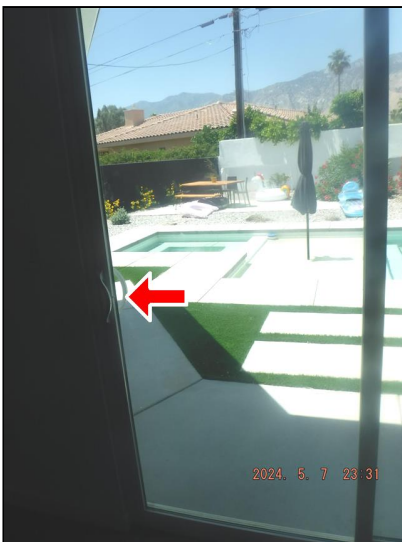
5.4 Item 3(Picture) Living room sliding door
