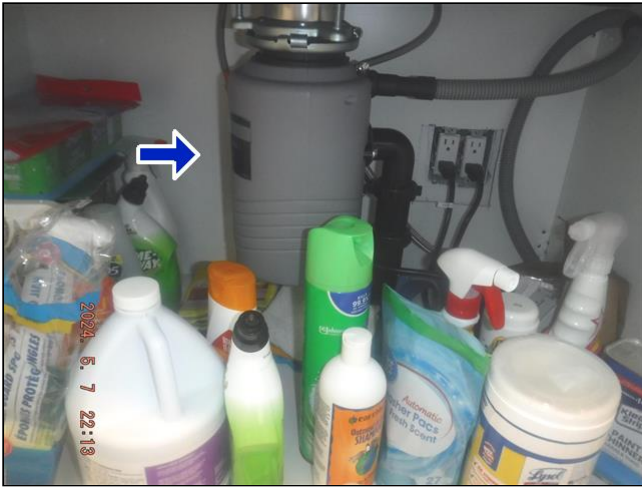
3.10 Item 1(Picture) Sink water valves location
